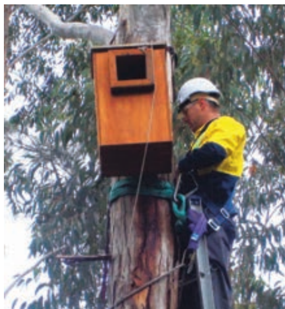
FIGURE 8.8: Nest box installation being carried out on the Sapphire to Woolgoolga project in Northern Region (Photo: RTA).
