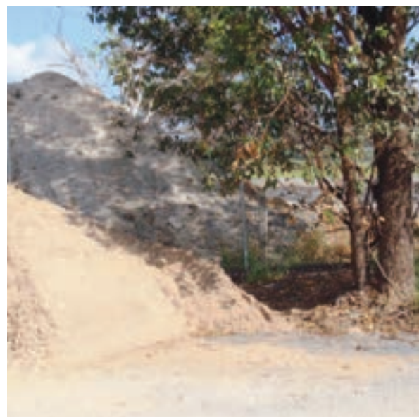
FIGURE 2.8: An example of poor practice. Equipment, vehicles and stockpiles should be outside the tree dripline or tree protection zone of trees (Photo: Rebecca Murray).
