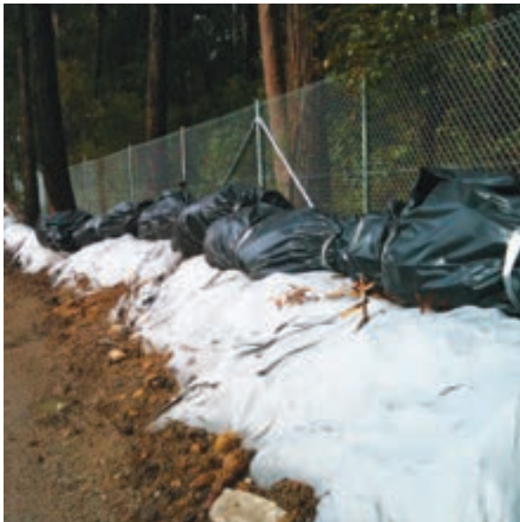
FIGURE 7.11: Removed vegetation was securely wrapped in black plastic bags before disposal to prevent the spread of the pathogen Myrtle rust on the M2 Upgrade, Sydney region (Photo: Nicholas Francesconi).
