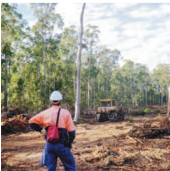
FIGURE 1: Clearing of native vegetation has the potential to impact on biodiversity. When clearing native vegetation, refer to Guide 4: Clearing of vegetation and removal of bushrock (Photo: RTA).
