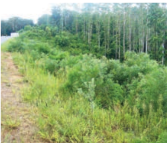
FIGURE 3.5: Seeding with native species on Bonville bypass has been successful, especially adjacent to the existing state forest where moist, sheltered conditions occur (Photo: Gareth Collins).
