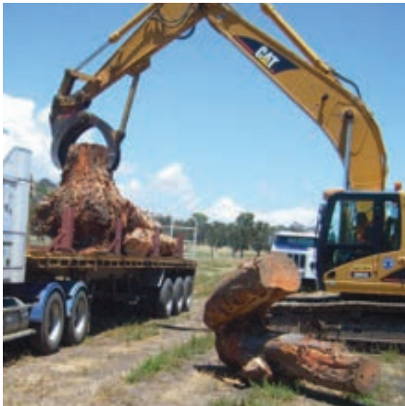
FIGURE 5.4: The RTA provided trees felled for the Hume Highway duplication project for the Murray River Resnagging project. Large logs were transported by truck from the road works site (Photo: M Casey, DPI).
