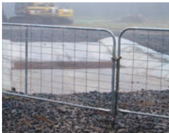
FIGURE 7.8: Wheel wash bay used at Sassafras during upgrades on Main Road 92 (Nowra to Nerriga) Southern Region. Vehicles drive onto the grid and are washed down. Water is contained under the grid (Photo: Julian Watson).
