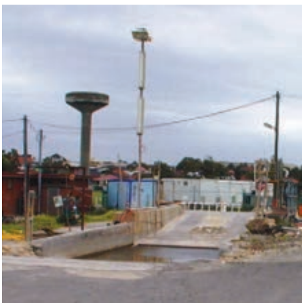
FIGURE 7.7: Wheel wash bay used at Tempe Reserve during construction of the Airport Link, Sydney Region. Most trucks drove through the wheel wash, but some vehicles needed to be scrubbed to ensure materials were not transported from site. The water depth was approximately 400mm, with a cattle grate underwater for solids to settle under (Photo: Leigh Trevitt).
