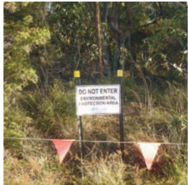
FIGURE 2.1: Exclusion fencing showing an environmentally sensitive area on the Hunter Expressway (Photo: Josie Stokes).
