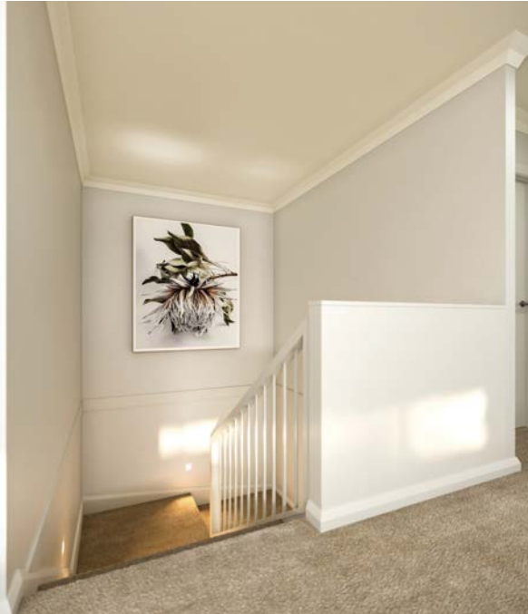
Half-height plasterboard stair wall with painted timber capping
